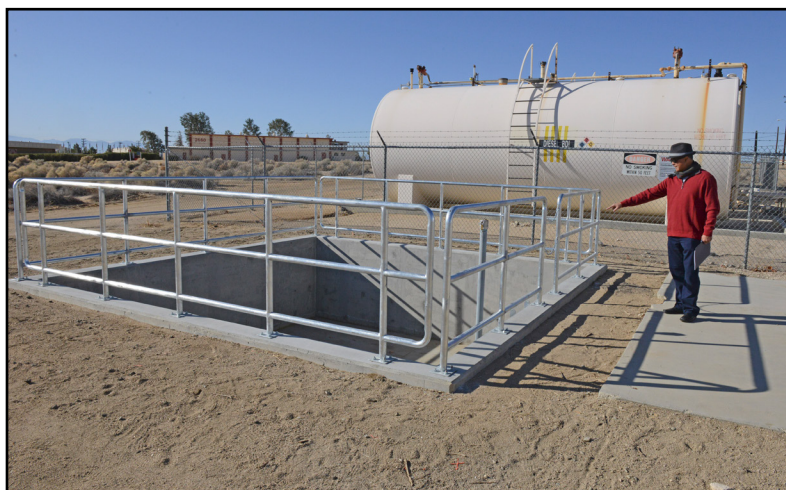
Jose Delavega, 412th Civil Engineer Group civil engineer, stands next to a new isolation pit to contain accidental fuel spills at the fuel transfer area at the main base military gas station Feb. 26. (U.S. Air Force photo by Kenji Thuloweit)
