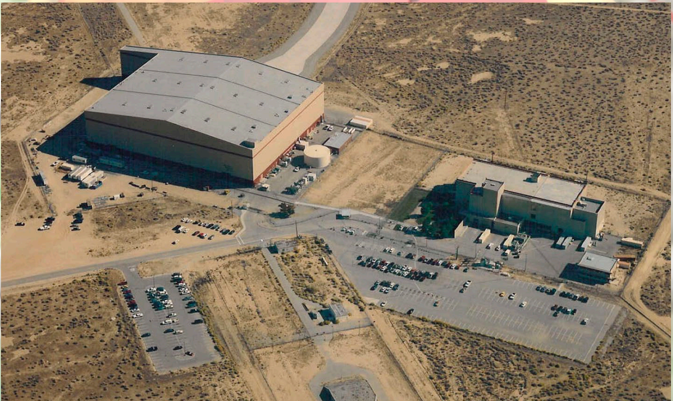
The BAF at the Avionics Test and Integration Complex (ATIC)
