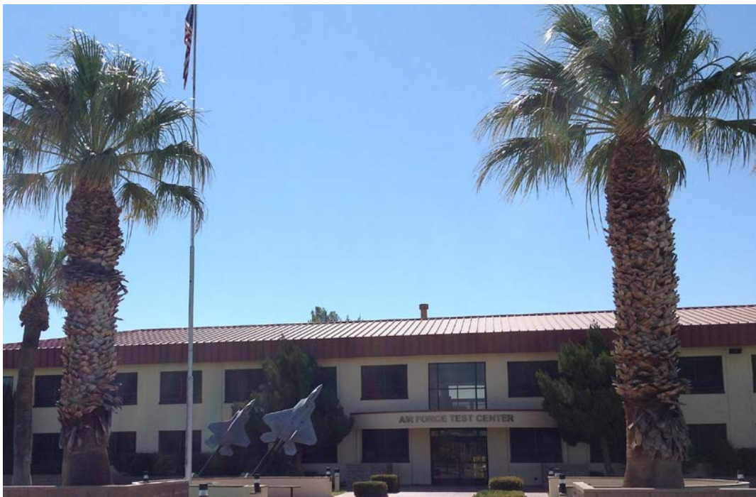
Air Force Test Center Headquarters, Building 1, Edwards Air Force Base, Calif.
